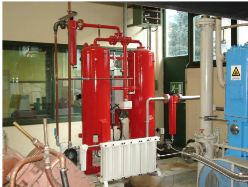
Slika 5: Sušilnik in filter
