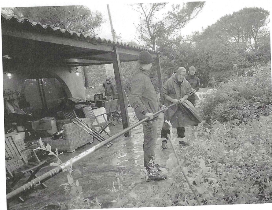
Figure 12 — Assembling 40-meter verticals.
